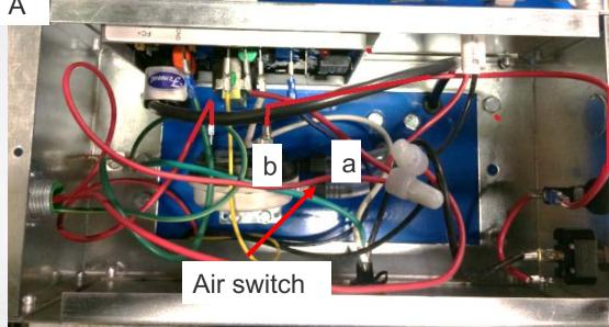
If voltage is present at "a" but not "b", you either have too much static pressure and the switch does not have enough airflow to close (see fan heater combination charts), or the switch is defective
