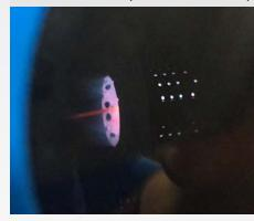
2. Not enough air: Take a look at the flame through the viewing window. If the flame has yellowish/orange tongues and is burning a bit further out the burner body, that is an indication that there is not enough air.
